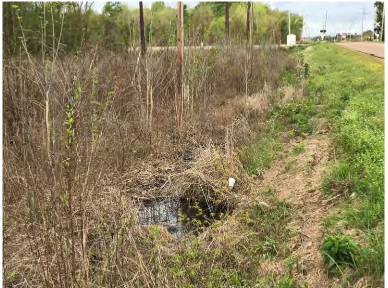
Photo taken looking west at existing road toe.
